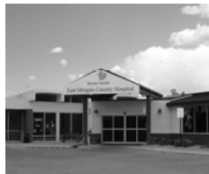
East Morgan County Hospital, a CAH in Colorado
