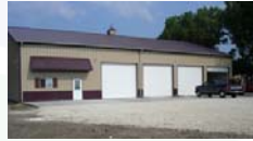
Rural fire station, northeast Kansas
