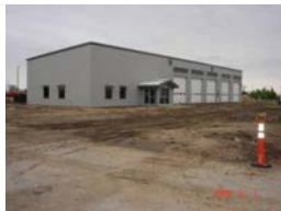
Greensburg Road & Bridge Project
